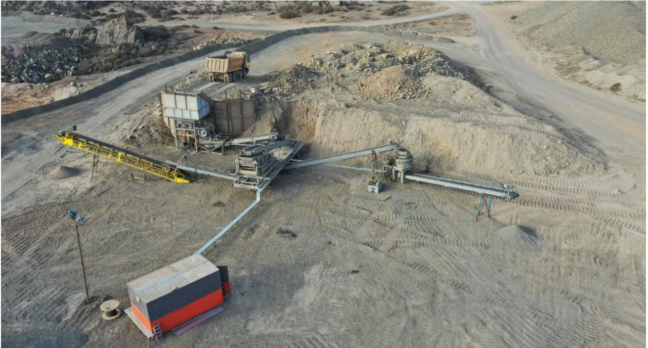
Image 2: MTN's fixed two-stage crushing plant with primary and secondary crushing units
