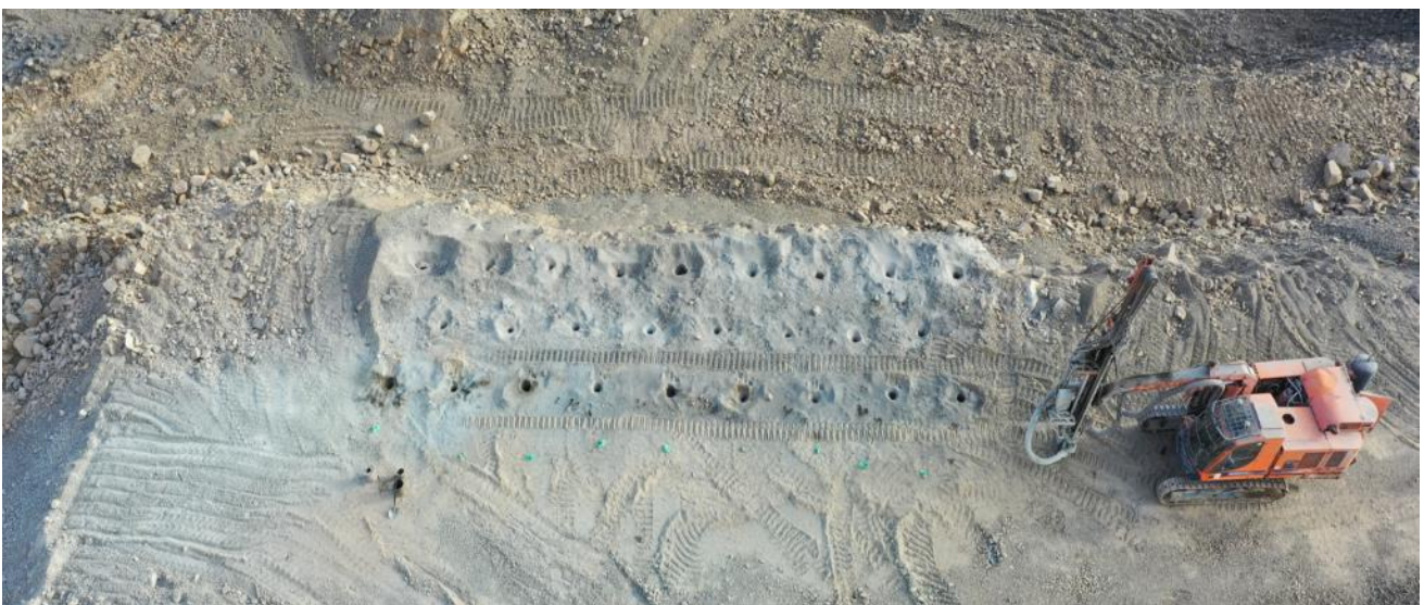
Image 3: Several of the 199 holes being drilled ahead of the blasting program
