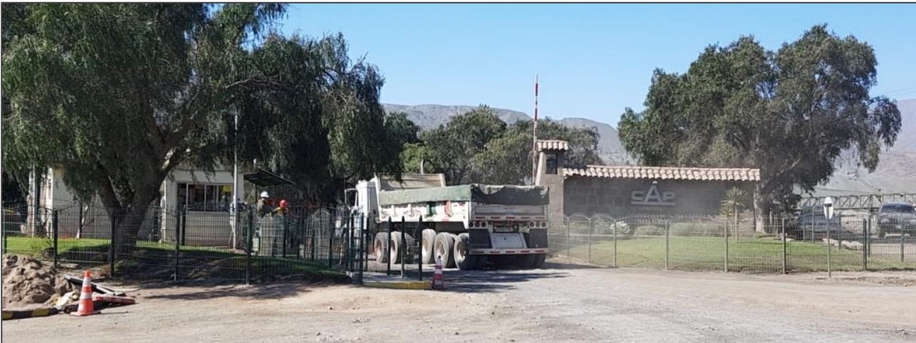
Figure 2 – Freehill magnetite concentrate being delivered into CAP Romeral iron ore pellet feed plant
