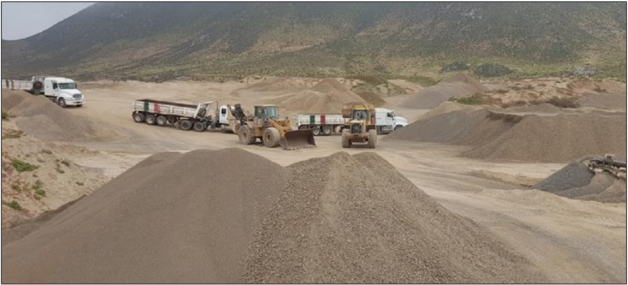
Figure 1 - Magnetite concentrates being loaded into trucks for delivery to CAP Romeral pellet plant 30km south of the mine site
